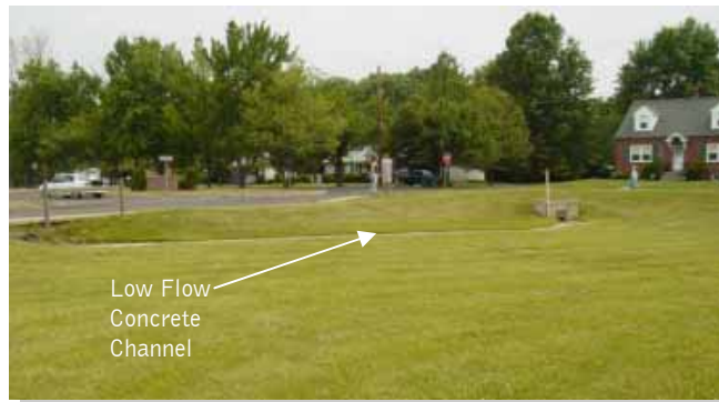
A conventional detention basin with a low flow concrete channel
