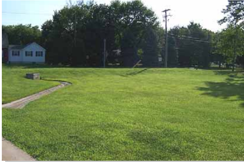
West Rockhill Elementary School conventional stormwater detention basin showing concrete low flow channel leading to outlet structure near Washington Avenue.
