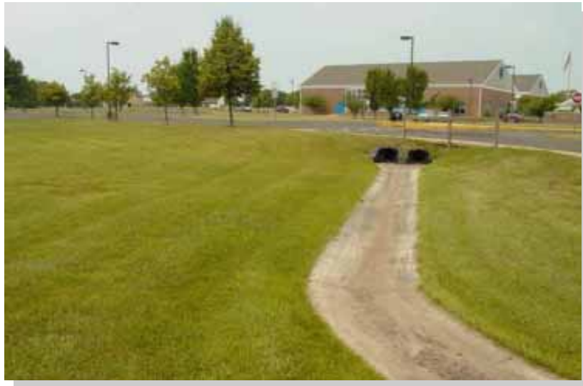
West Rockhill Elementary School conventional stormwater detention basin showing inlet into basin and adjacent impervious surface areas.
